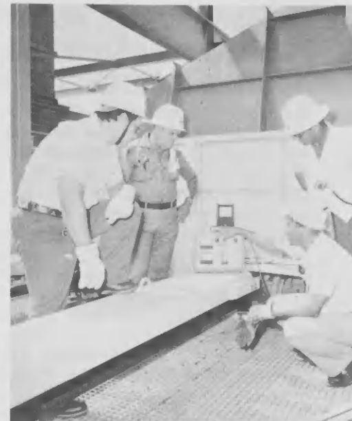
Members of the Energy Conservation Team (Leonard Peterson, Emiliano Trimon, Eddy Laclé, Edgar Maduro (foreground) measure oxygen content with a portable oxygen analyzer at the top of the furnace.
